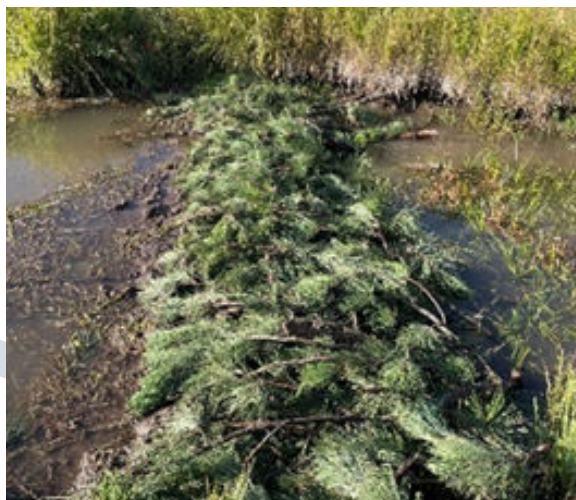
This photo shows a completed beaver dam analogue (BDA)
