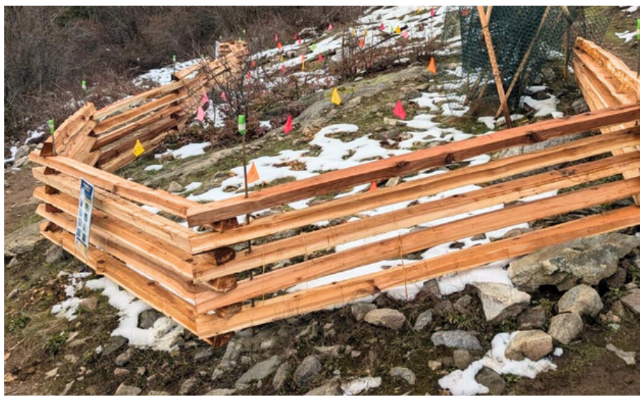
Split rail cedar fence installed at Dove Hill native plant restoration site, November 2024.
