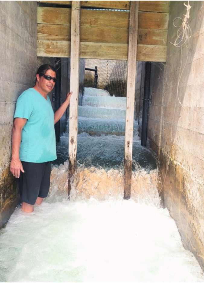
Photo: A fish ladder at the Okanagan Lake Dam as part of a ntytyix Passage Project was installed
