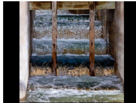
Okanagan Lake Dam Fishway Entrance
