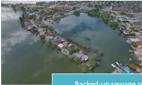
Backed-up sewage system
