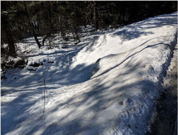
Stop 2: New culvert replaced on downstream side of Hedley Road (RL)
