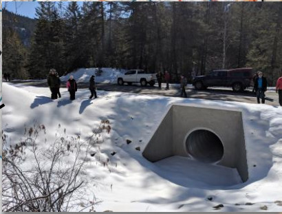
Stop 2: Flooded creeks on Old Hedley Rd.
