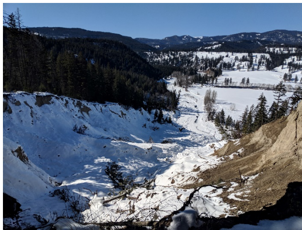
Stop 1: View west down the path of the landslide (RL)
