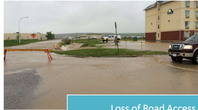
Loss of Road Access
