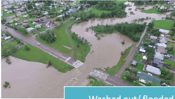
Washed out/ flooded roads
