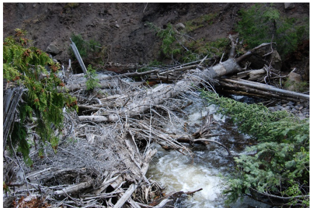
Stop 8: Close-up of debris in Bouleau Creek bridge.
