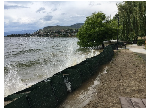
Figure 11: High water levels on Okanagan Lake (Source: WFN).
