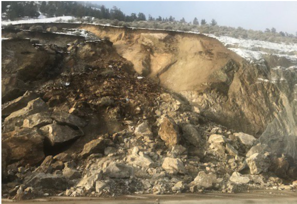
Figure 17: Rock fall on Highway 97 (Source: MOTI).
