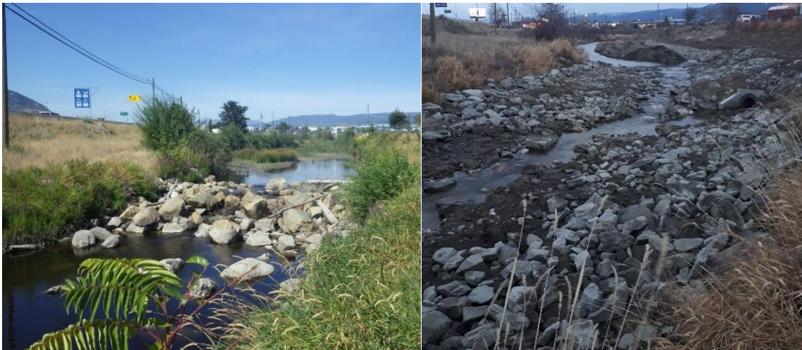
Ellis weir in 2016 (left) and fish passable riffle in 2018 (right)
