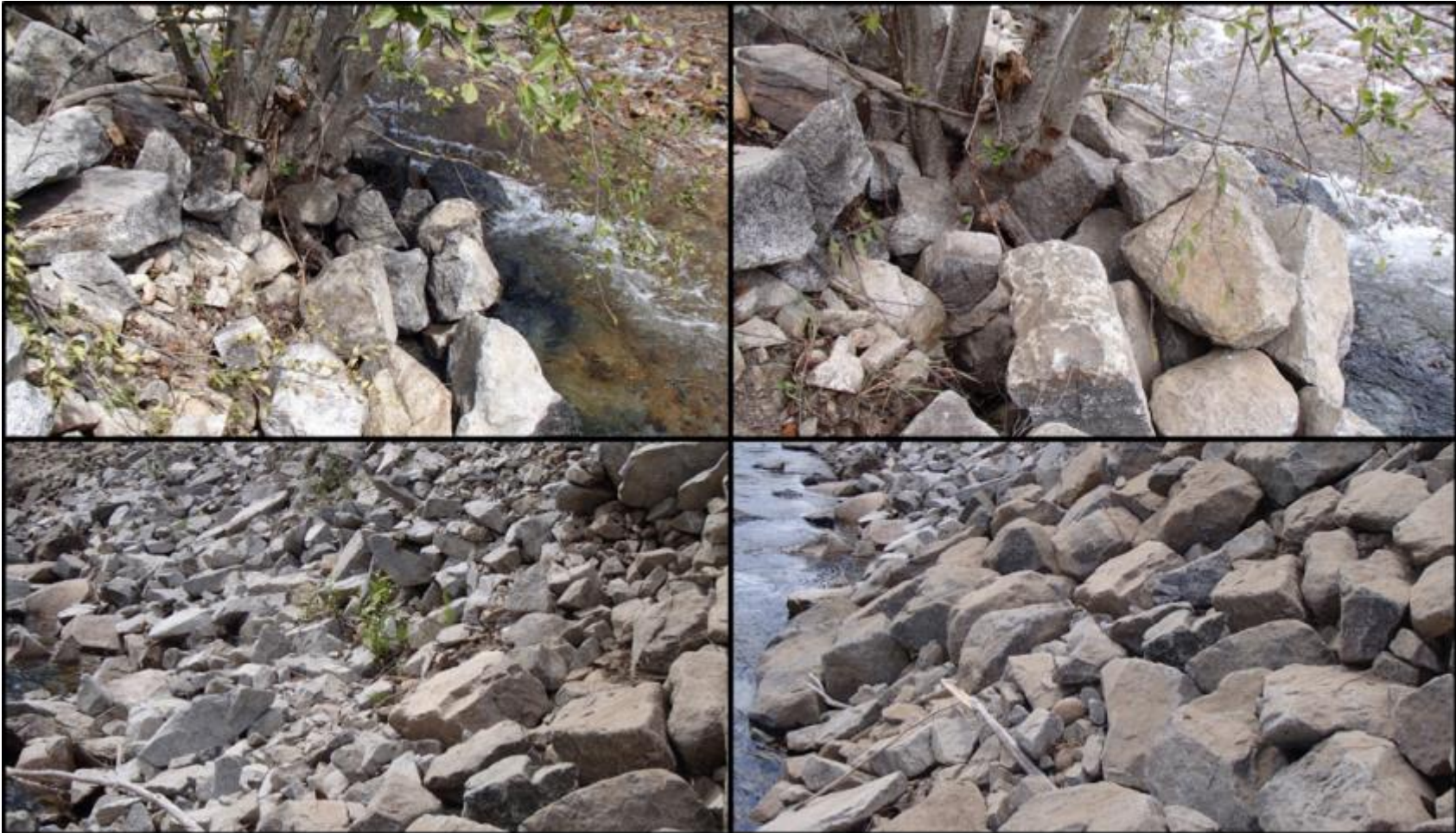
Figure 7. (Top) Before and after comparison of minor bank reinforcement along the toe of the rip-rap bank at Pass Creek. (Bottom) Before and after comparison of target bank stabilization conducted along the rip-bank at Pass Creek. Additional rock was placed at the bottom of this slope to support the top of the rip-rap bank; transforming it from a concaved bank to a 45 degree slope. (all pictures taken by Evan Smith, Okanagan Nation Alliance, July 2015).
