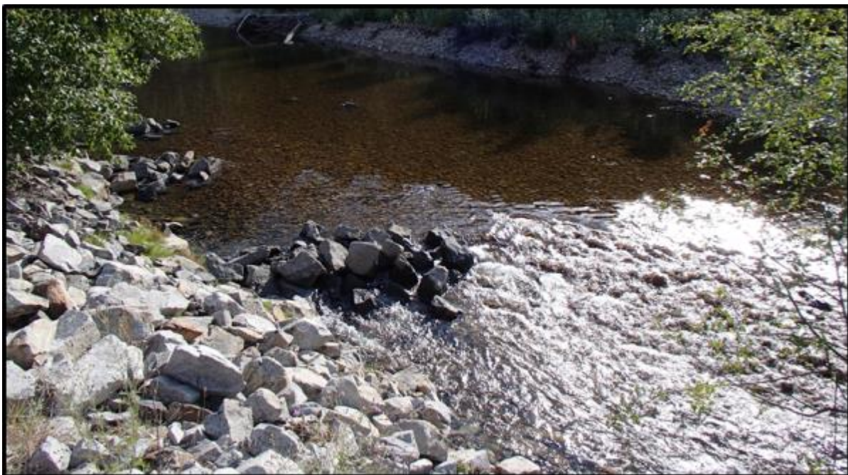
Figure 9. Rock structures created along the rip-rap bank in the Pass Creek Regional Exhibition Grounds creating pools and cover for rainbow fry (picture taken by Evan Smith, Okanagan Nation Alliance, July 2015).
